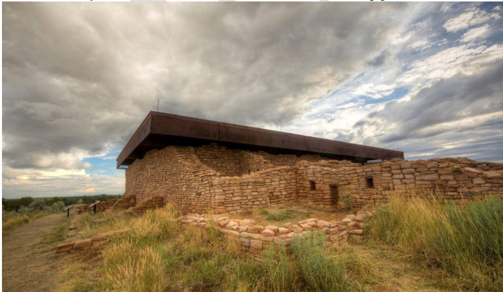
Photo 5. Lowry Pueblo (The metal roof was constructed to help preserve the site.)
